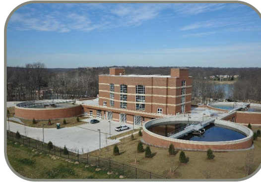
Residuals Management Project
