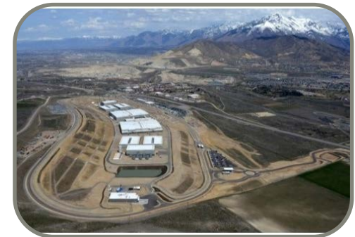
Utah Data Center
