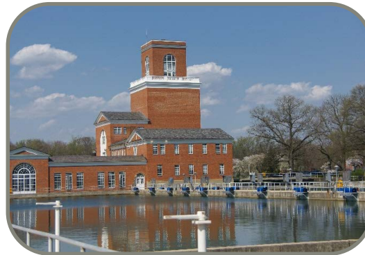
Dalecarlia Water Treatment Plant
