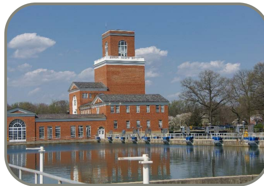
Dalecarlia Water Treatment Plant
