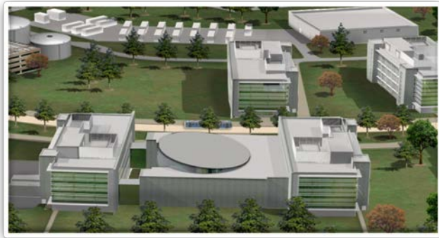
Joint Operations Center
