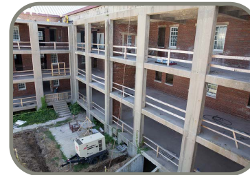
Hale Hall Renovation Fort Meade, MD
