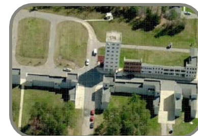
J.J. Rowley Training Center Upgrades
