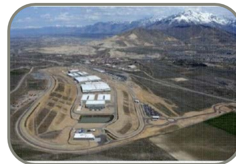
Utah Data Center
