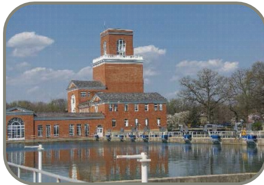
Dalecarlia Water Treatment Plant
