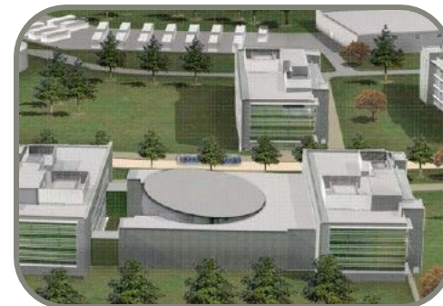
Joint Operations Center
