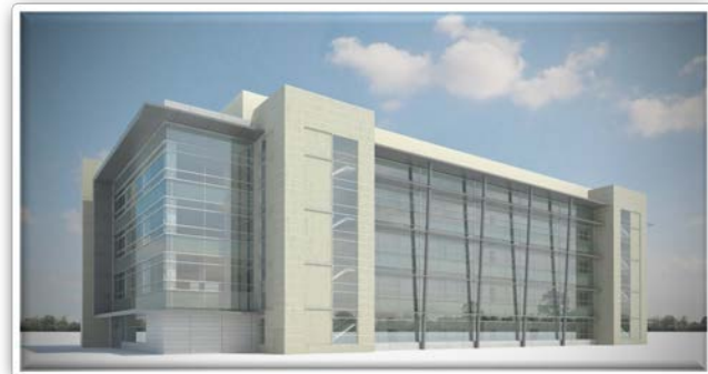
East Campus Building Marine Corps
