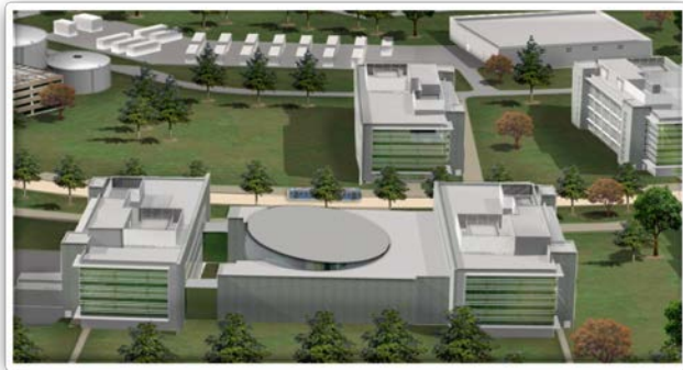
Joint Operations Center
