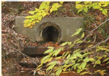
Stormwater outfall at Whitsons Creek
