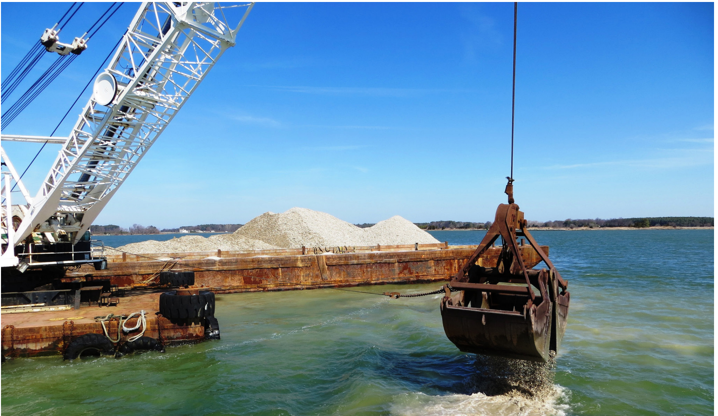
The U.S. Army Corps of Engineers, Baltimore District, places shell to restore oyster reefs in the Chesapeake Bay tributary of Harris Creek, April 1, 2015.
