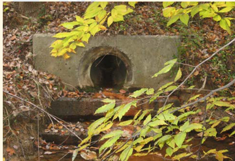
Stormwater outfall at Whitsons Creek
