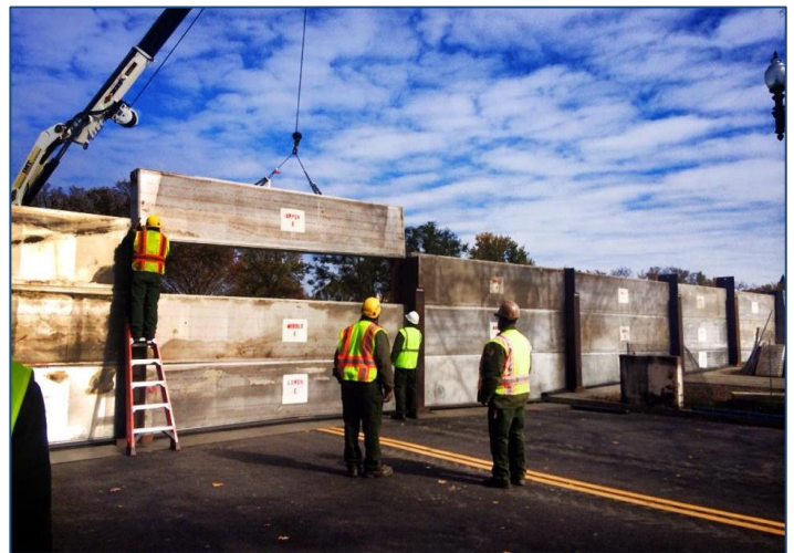
Photographs from the U.S. Army Corps of Engineers of the 17 th Street Closure Trial Installation on 10/31/2014
