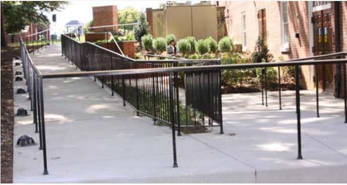
The Baltimore District design team solved several key problems with an Americans with Disabilities-compliant ramp that provides easy access for both the main chapel and reception area. The ramp included benches, for personal reflection, that face Arlington Cemetery to the left.
