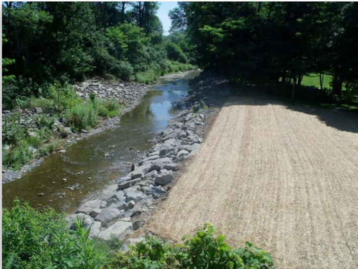
Completed rehabilitation work under PL 84-99 in Bainbridge, N.Y. The construction project was in response to severe flooding from Tropical Storm Lee in September 2011. (Courtesy photo)
