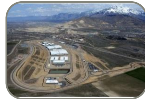
Utah Data Center
