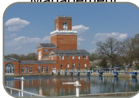
Dalecarlia Water Treatment Plant
