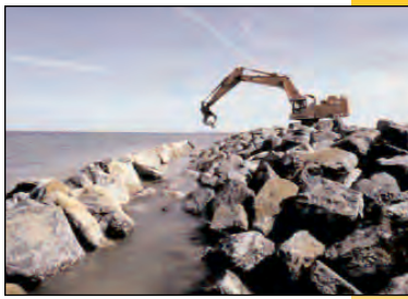
Behind reinforced dikes built around the perimeter of the Island, workers offload the dredged material from barges. It is sent through a pipeline to the appropriate place on the island for use in habitat development.
