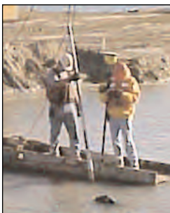
Surveying for perimeter dike construction.
