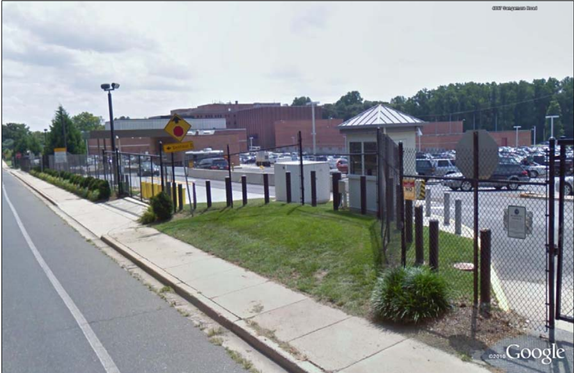
Figure 4-6: View of the Sumner Site from Sangamore Road
