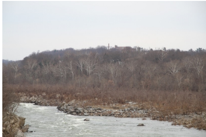
Figure 12: Existing view of ICC-B from Chain Bridge (Image date: unknown)
