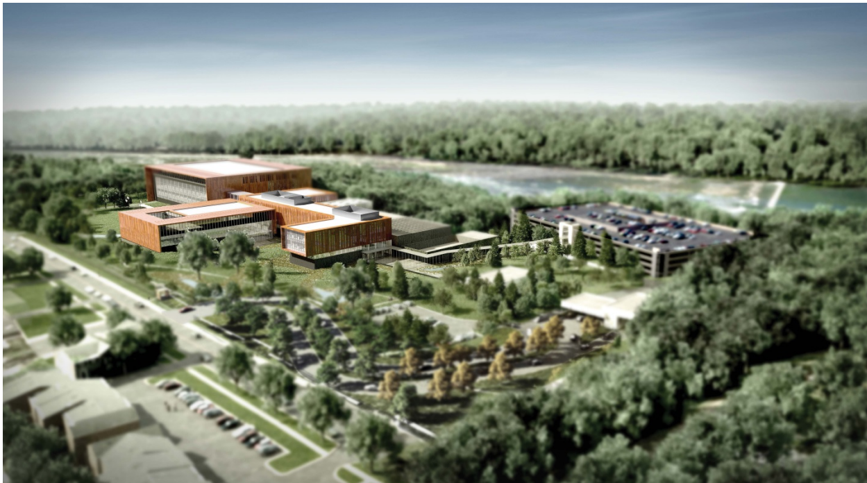
Figure 16: Illustrated overview of the completed ICC-B Campus Looking southwest (Image date: June 6, 2013)
