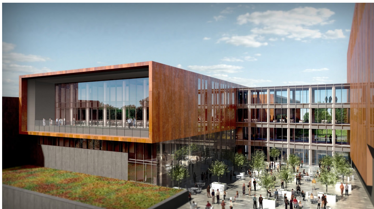
Figure 7: View of Centrum – South Wing (green roof, cafeteria, and Assembly Court) Looking northeast toward Sangamore Road (Image date: June 21, 2013)
