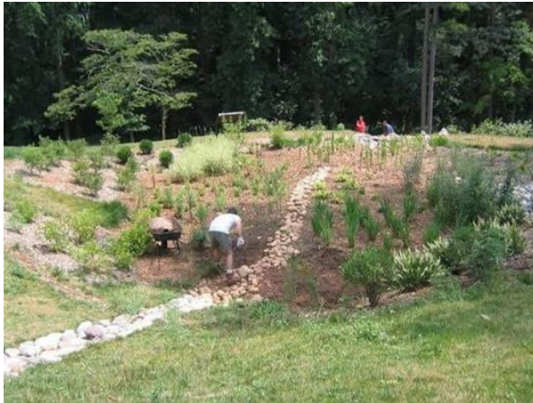
Figure 16: Example of a micro-bioretention area.
