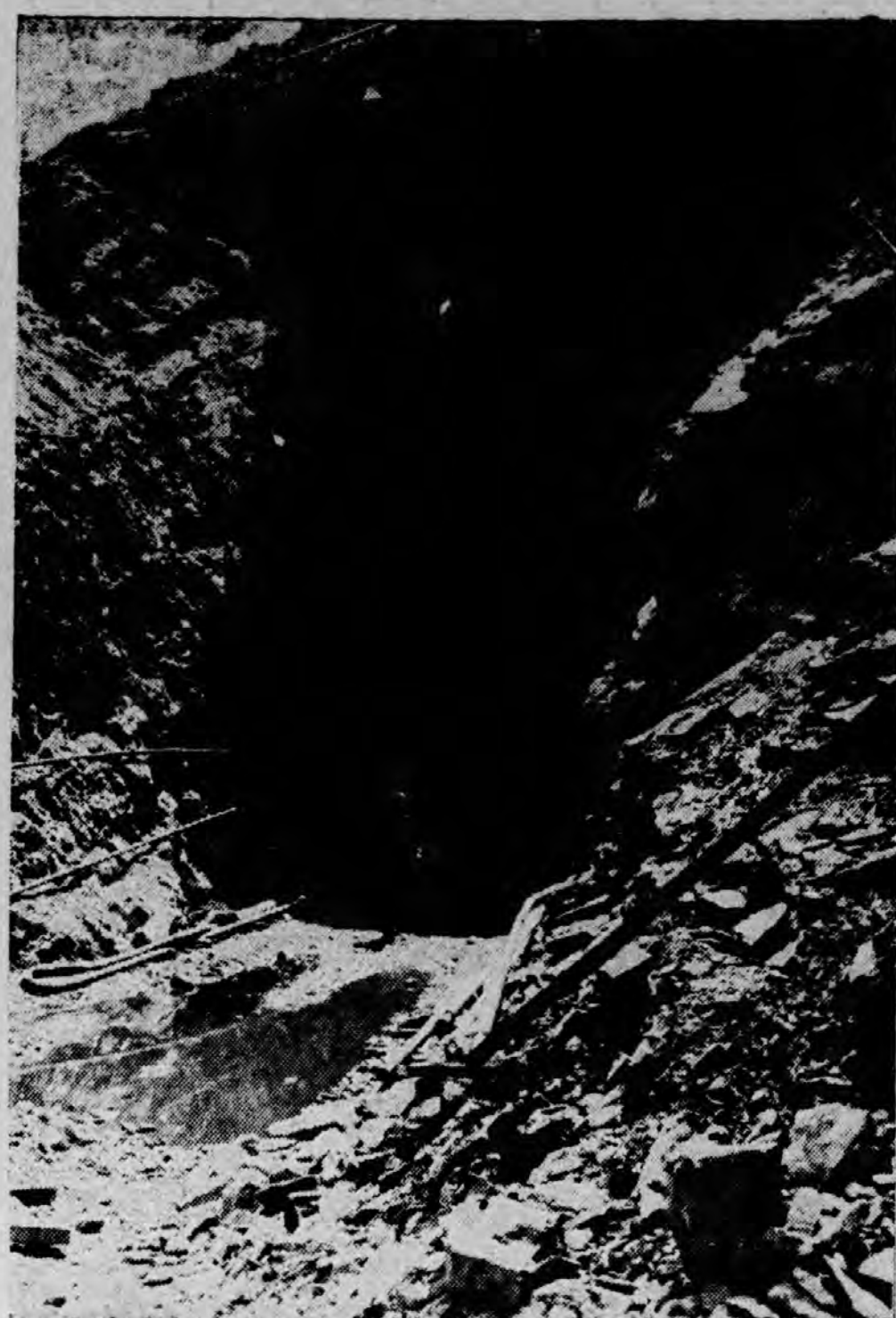
This picture shows the one end of the tunnel. This is being cut through a hillside and will be about 360 feet in length. This tunnel, when finished, will be solid concrete.
