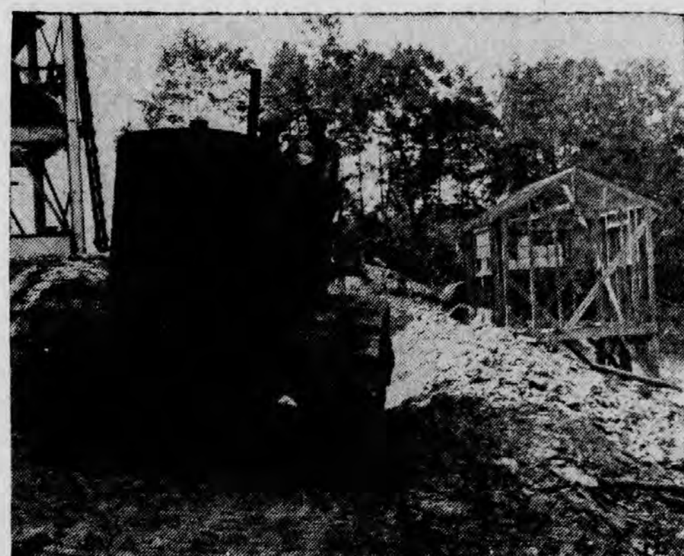
—Photos By The Gazette And Daily This is just one of the many tractors the U. S. War department has at the construction scene.
