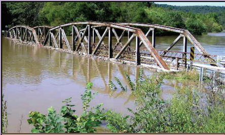
Old Weaver Falls Bridge
