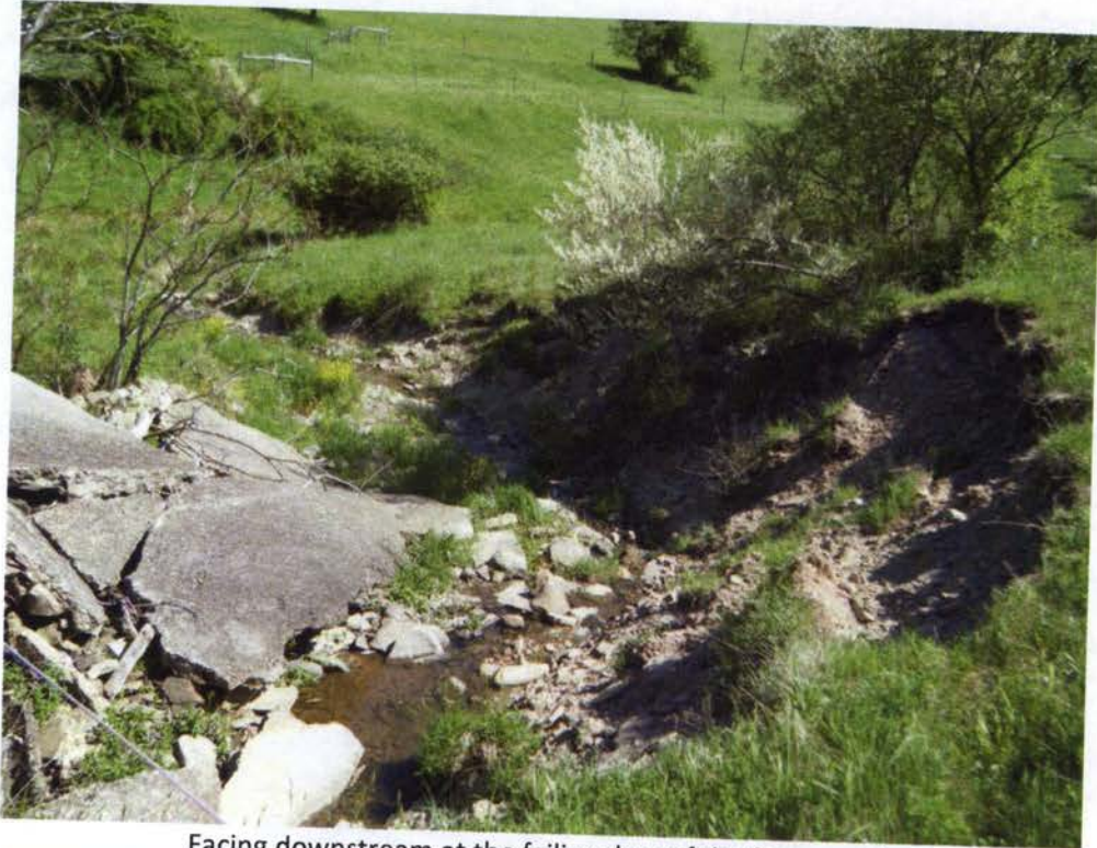
Facing downstream at the failing dam of the farm pond.
