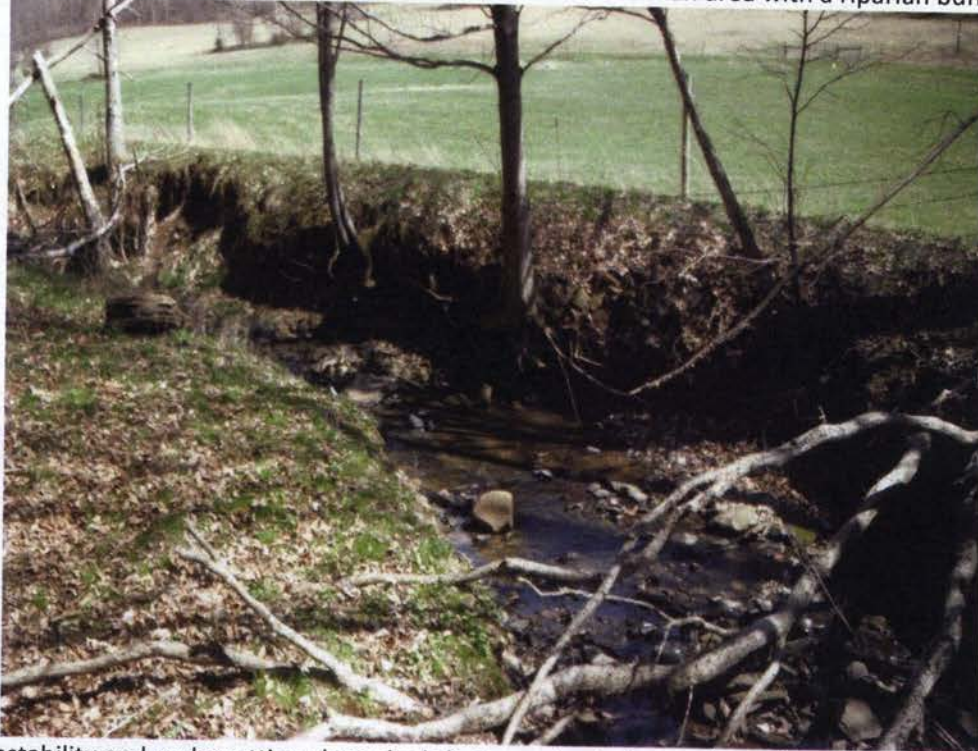
Bank instability and undercutting along the left stream bank due to channel migration and a lack of riparian buffer.
