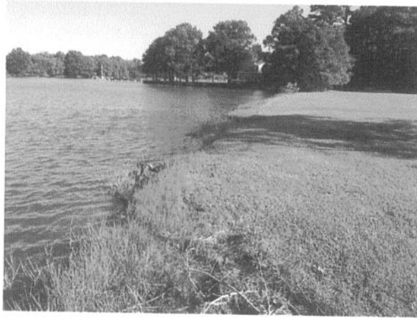
Project Site Looking North
