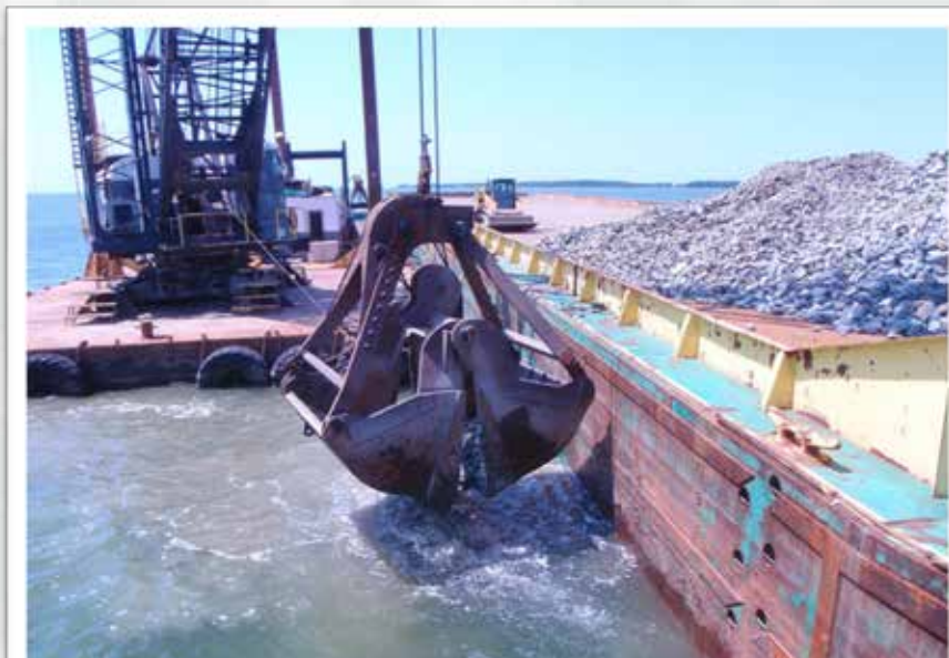
Placing Oyster Substrate in Harris Creek
