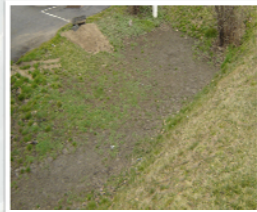
Existing Bio-Retention Facility
