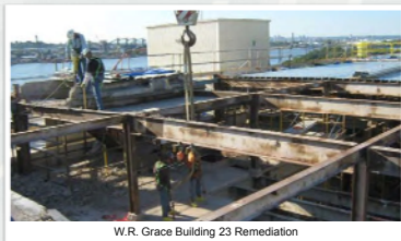
W.R. Grace Building 23 Remediation
