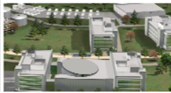
Joint Operations Center
