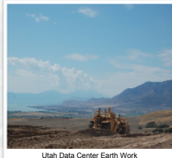
Utah Data Center Earth Work
