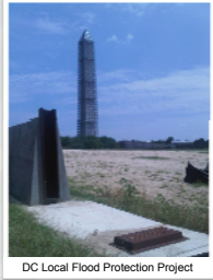
DC Local Flood Protection Project
