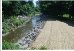
Bainbridge, N.Y. PL84-99 Repairs
