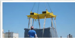
W.R. Grace Building 23 Remediation
