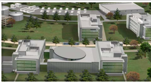
Joint Operations Center
