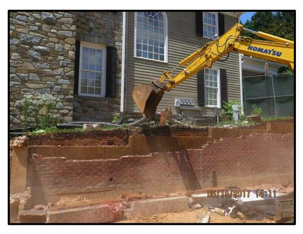
Mechanical excavation has been used where possible, for demolition of the retaining wall and to remove backfill placed behind the retaining wall during the prior arsenic removal efforts at the site.
