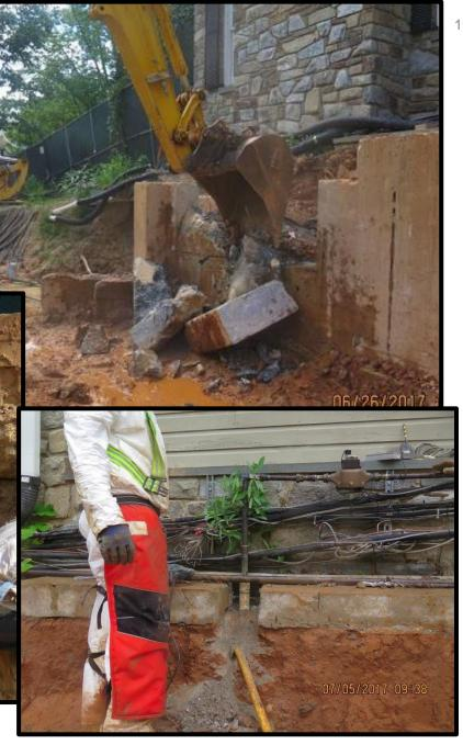
Rubble from the demolished retaining wall where CACM or AUES debris was recovered, is broken into small pieces so it can also be placed into drums for disposal.
