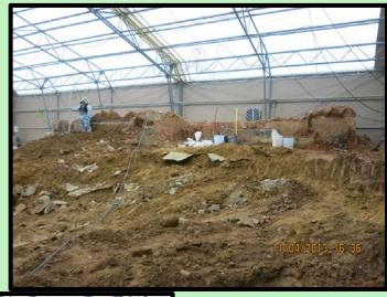
Removal of the hardscape (i.e. retaining wall and stairs) in the front yard, as well as a small portion of the front basement wall
