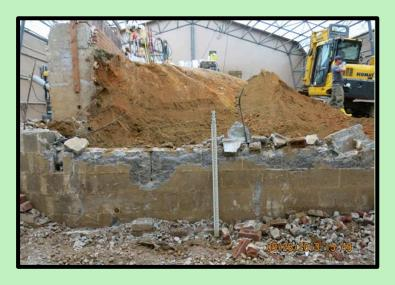
By mid-October, the crew completed the removal of the retaining wall between the driveway and the front yard to provide unobstructed access to the front yard area
