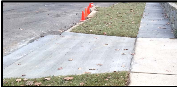
Restored driveway apron and sidewalk.
