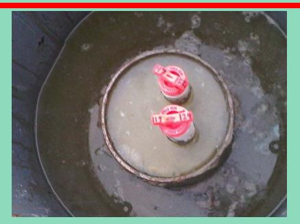
Two well screens were placed at approximately 120' and 150' which will allow sampling from those specific depths within the well.
