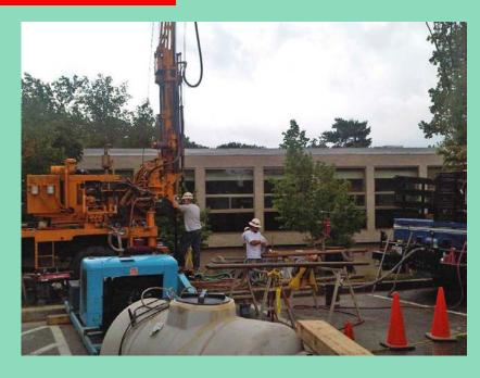
Purpose: Help characterize the extent of vertical perchlorate contamination in the area.
