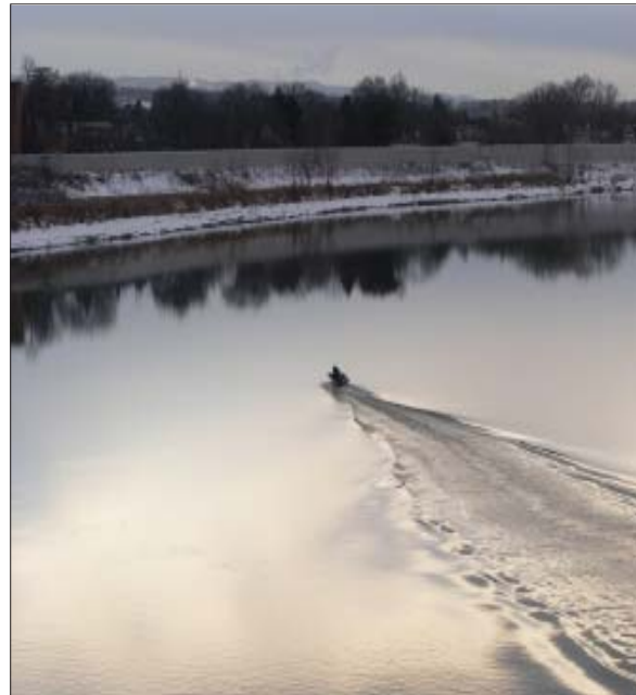
A boater nears the floodwall at Wilkes-Barre.
