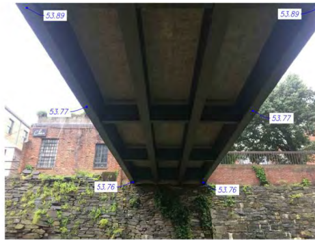
BOTTOM OF BRIDGE BEAMS
