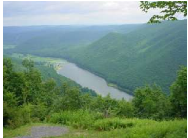
Photo: U.S Army Corps of Engineers
