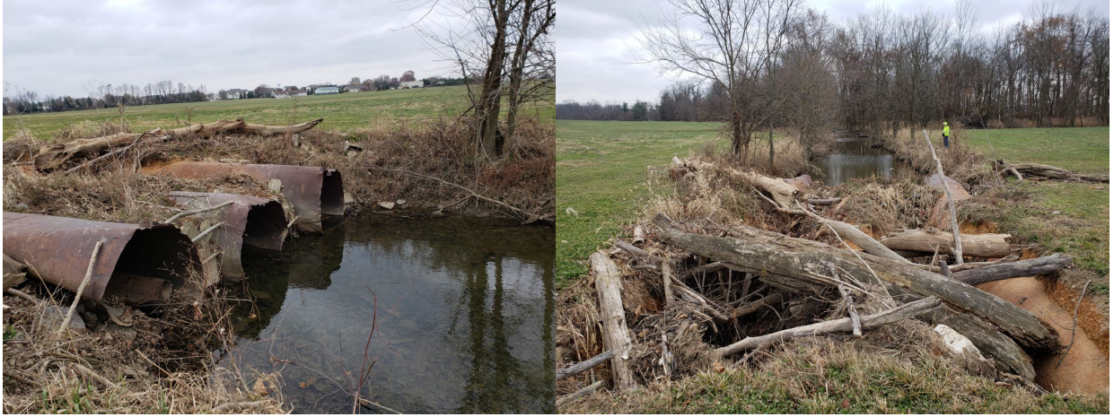
Figure 3: Photographs of the upstream end of the pipes. Note the structural condition of the pipes.
