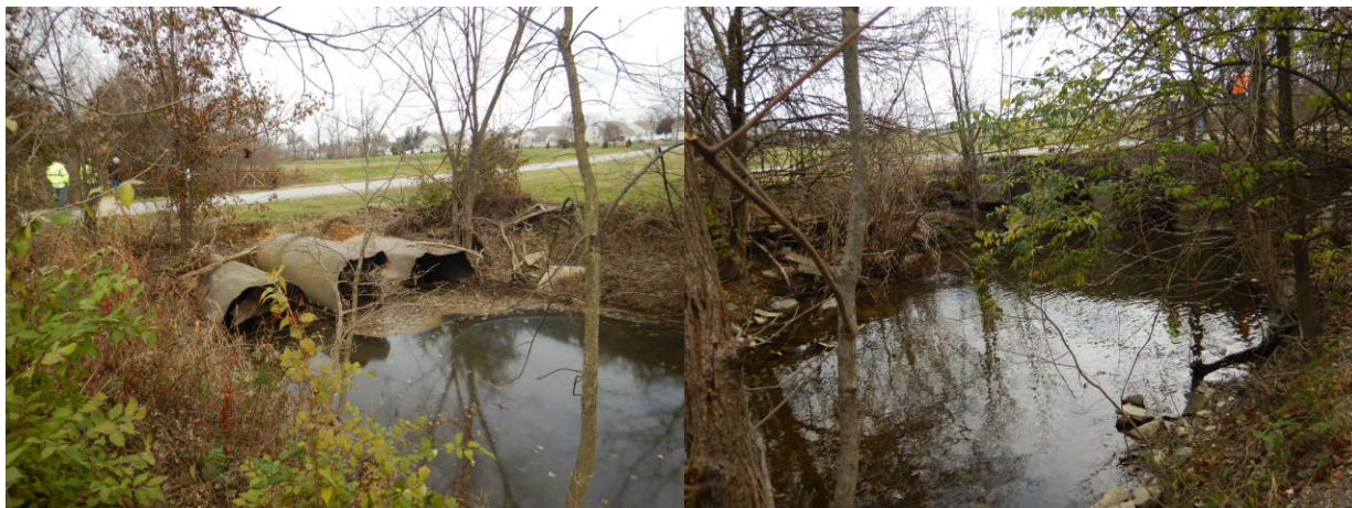
Figure 6: Inflow (left photograph) and outfall of pipes going under the bridge. Note poor condition of pipes (left picture).
