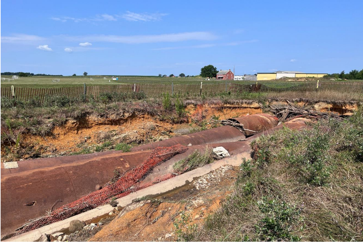
Photo 19. Pipes within Plum Creek showing debris and fill profile. Facing northwest.
