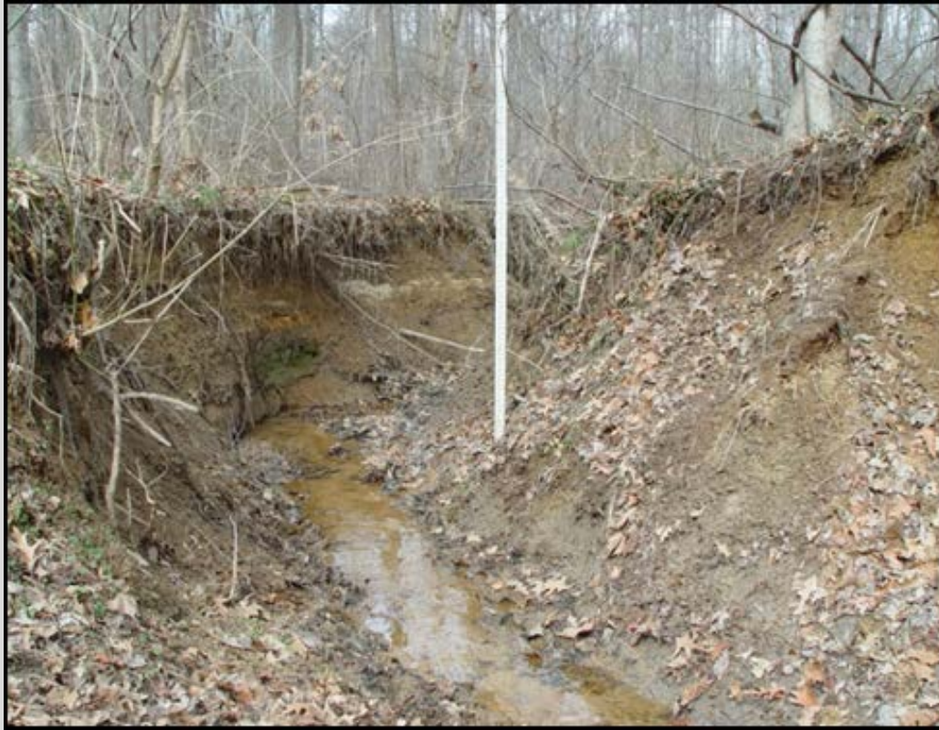
Photo 3. Example of Degradation
