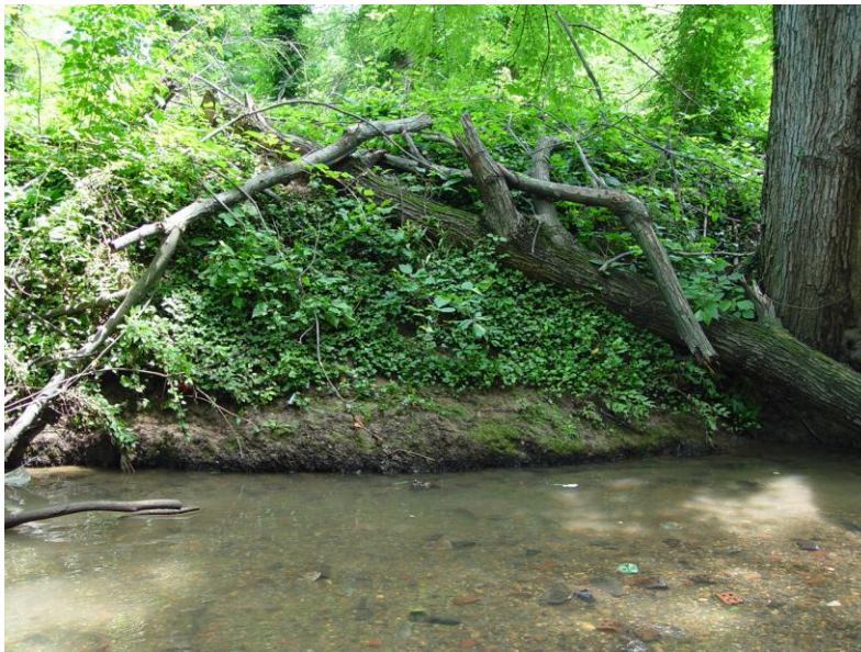
Figure10.Suspended log bank protection.
