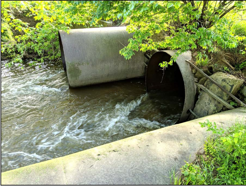
Photo 4 (5/6/2019) Viewing culvert outfall and downstream portion of the project area.
