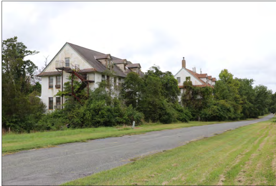
Dilapidated facilities along Poultry Road have been vacant for over 10 years.
