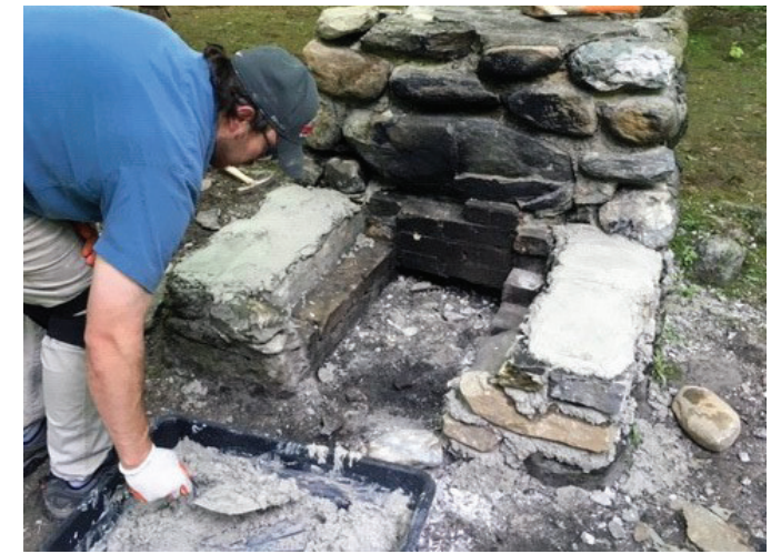
Ethan Bean, Baltimore District archaeologist, applies a mortar wash to the arms of a stone fireplace in Smuggler’s Notch State Park, Vermont, June 2019. (Courtesy photo)
