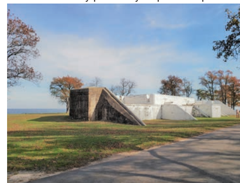
Battery Hartshorne at Fort Smallwood Park, Nov. 10, 2019.
