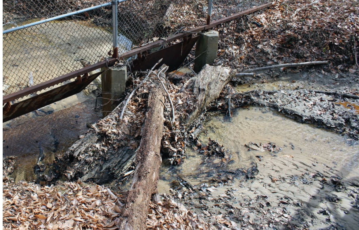
Logs and debris lodge open swing gates, creating a potential security concern, on Joint Base Andrews in Prince George's County, Maryland, Feb. 19, 2019. (U.S. Army photo by Sarah Lazo)
