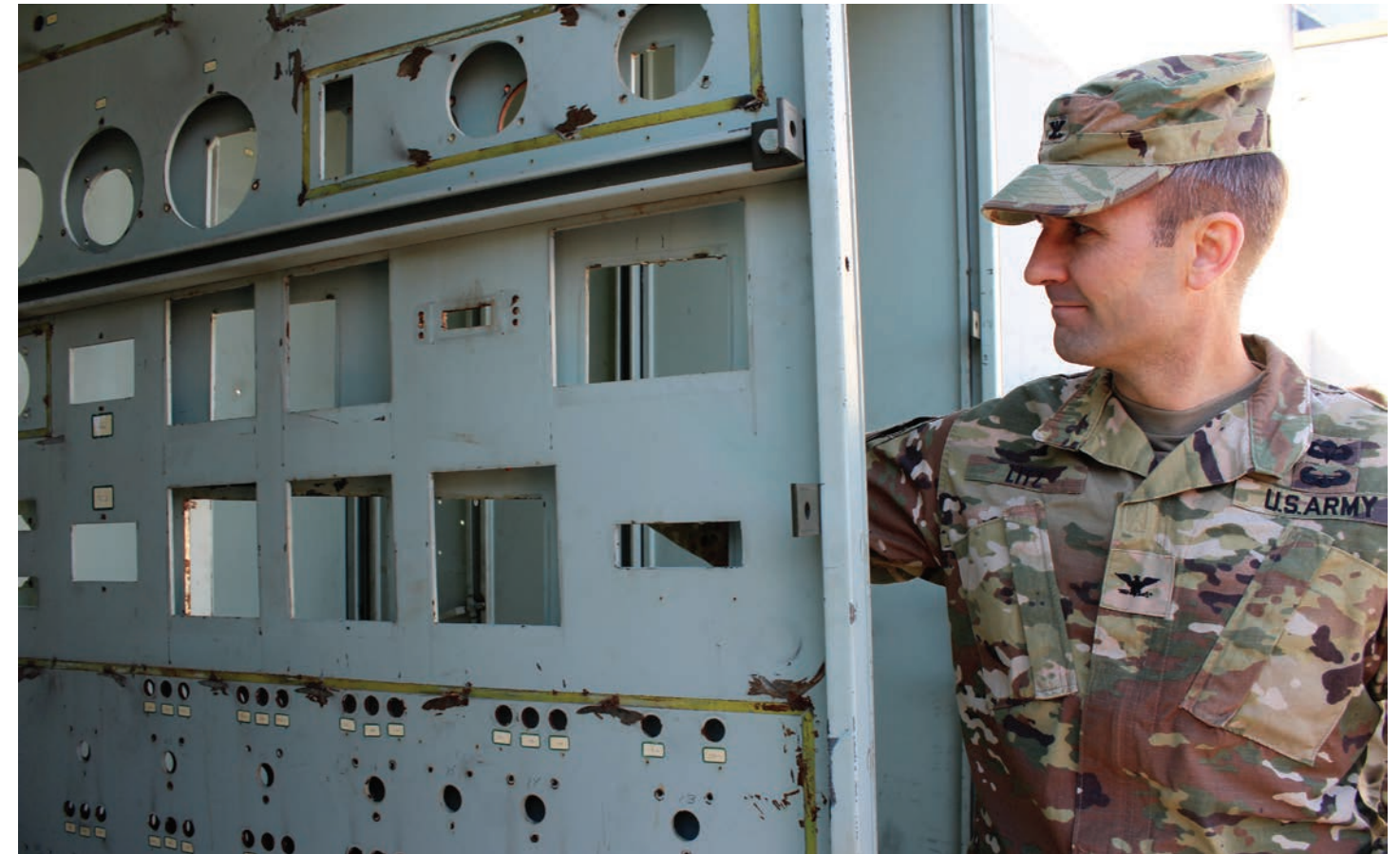
Col. John Litz, Baltimore District commander, looks at the SM-1A Deactivated Nuclear Power Plant's former control panel, located on Fort Greely, Alaska, April 24, 2019. Baltimore District, with its Radiological Center of Expertise, Fort Greely Garrison and Alaska District personnel are working closely on its decommissioning. (U.S. Army photo by Becca Nappi)
