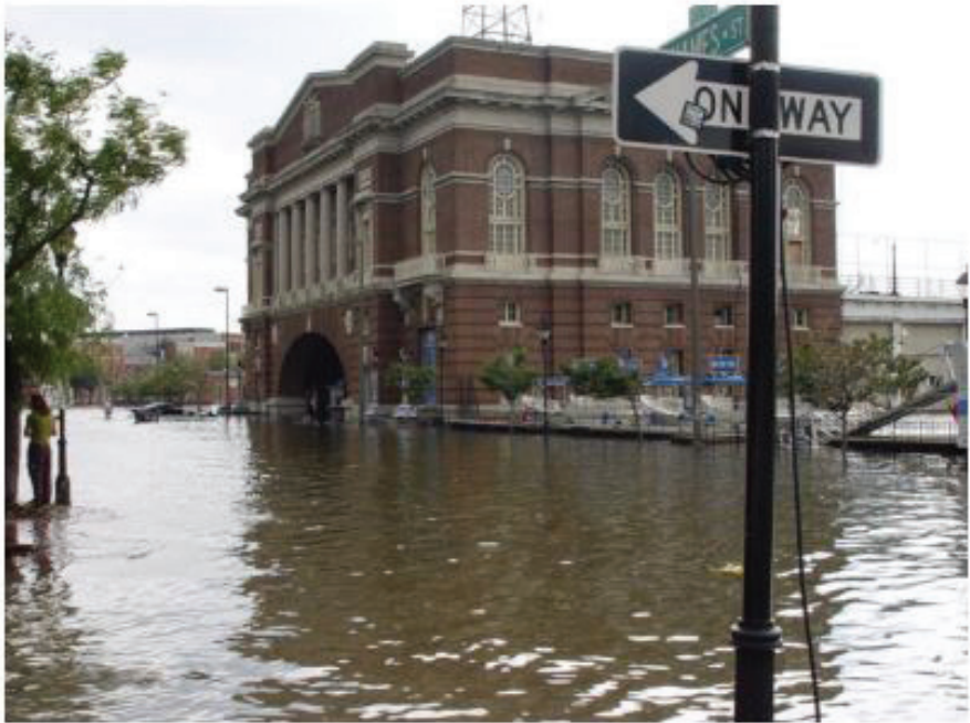
Fells Point Recreation Pier Flooding
