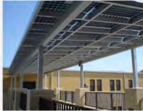
Pedestrian Photovoltaic Shade Structures
