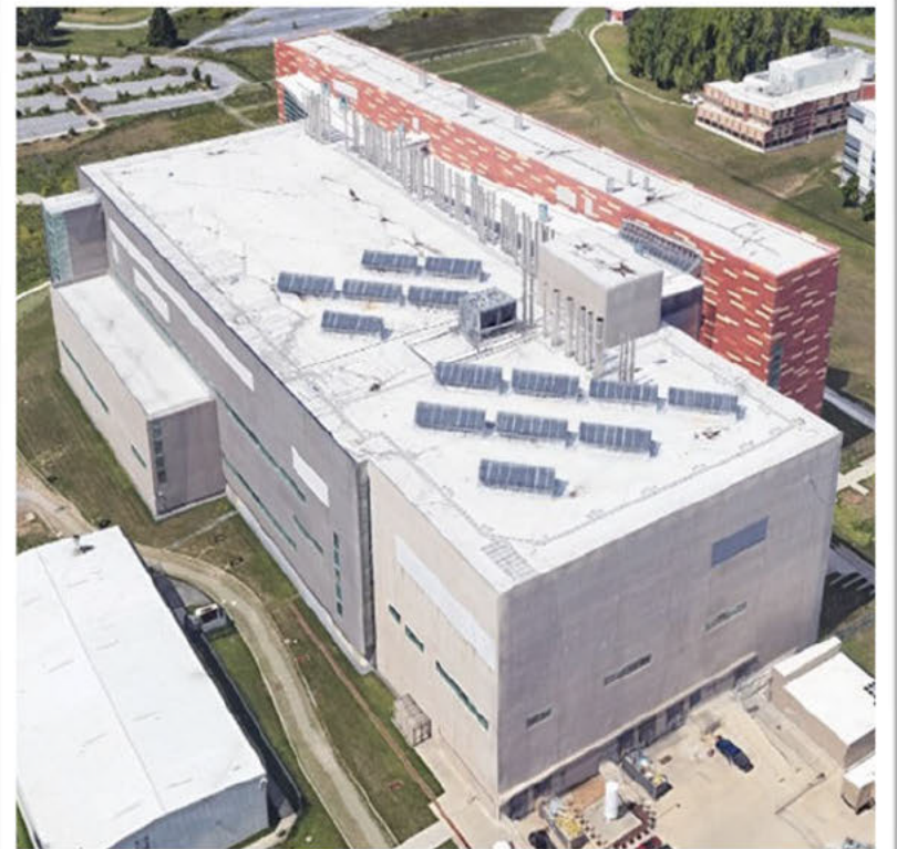
Photo 2 – Overview of Building (b) (7)(F) facing NW
