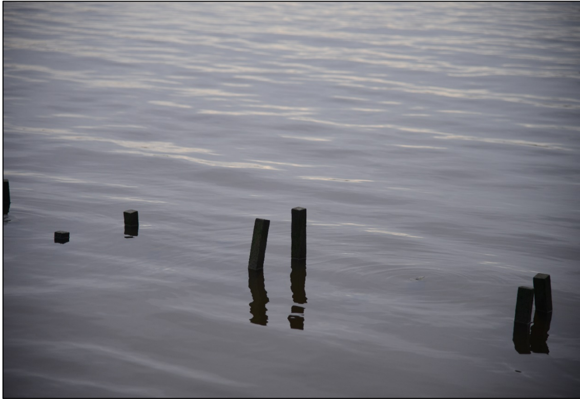
Figure 4. View showing square stakes used to hold coir logs in place. Square edges of stakes can result in chaffing of coir log cordage material holding logs in place.
