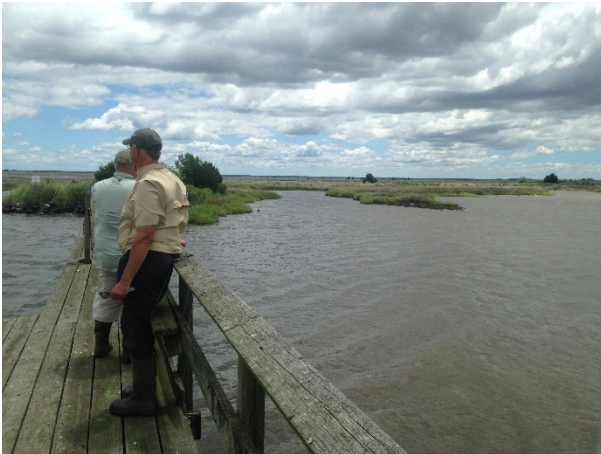
Figure 1 View looking east from water control structure. Proposed site includes marsh on the right of the photo. The embayment at center of photo is one of 3-5 to be filled by open water placement.
