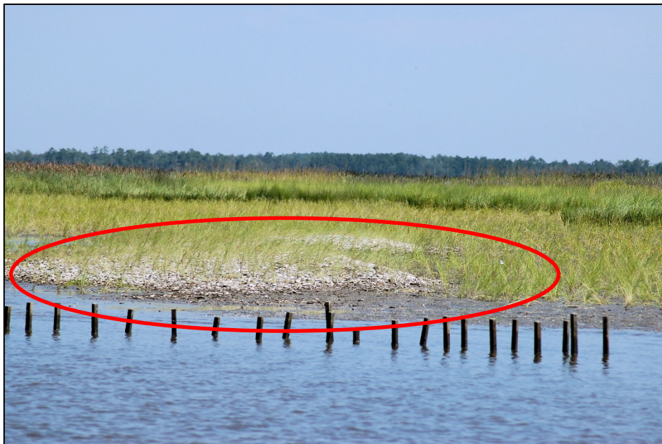
Figure 3a. 2017 view of backshore area planted behind coir log stakes.
