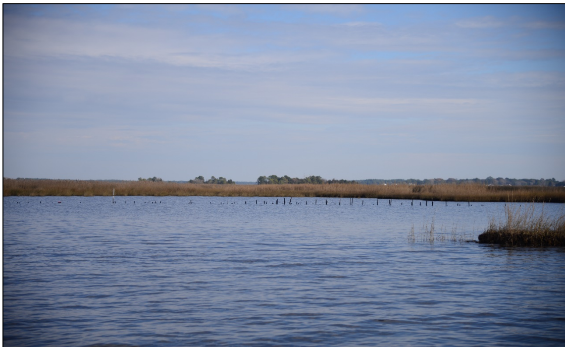
Figure 1. View looking east from southern end of project site; note exposed coir log stakes without coir logs attached.
