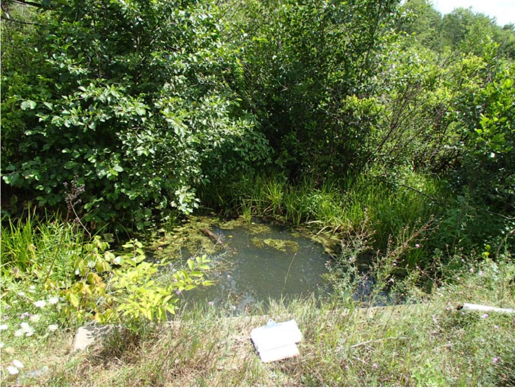
1 – CULVERT OUTLET, LOOKING DOWNSTREAM
