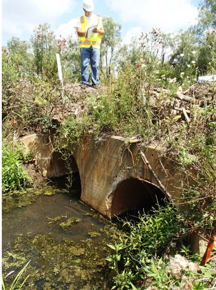
4 – CULVERT INLET AREA
