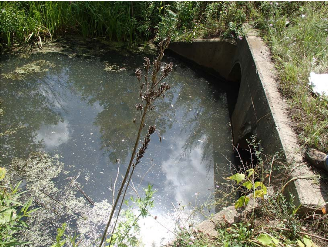
2 – CULVERT OUTLET AREA
