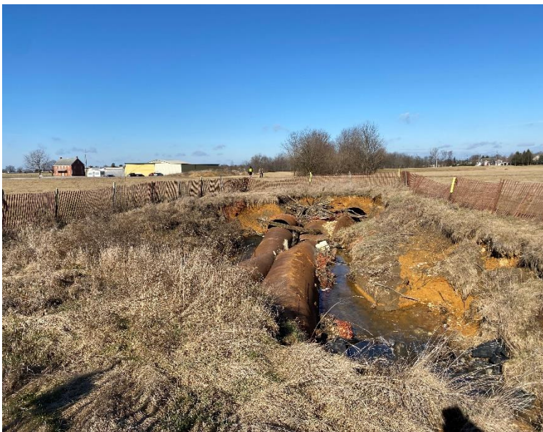
Photo 2: Plum Creek boilers/pipes facing west showing erosion in channel. Photo Source: USACE- Baltimore, January 2023
