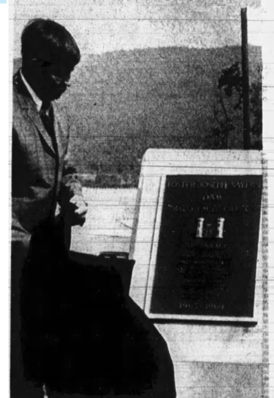
FOSTER JOSEPH SAYERS, JR., unveiling the plaque at the dedication of the Foster Joseph Sayers flood control dam at Blanchard, named in honor of his father. The dam was dedicated at ceremonies Wednesday under the auspices of the Susquehanna River Valley Flood Control Association, and the Chambers of Commerce of Lock Haven and Bellefonte.
