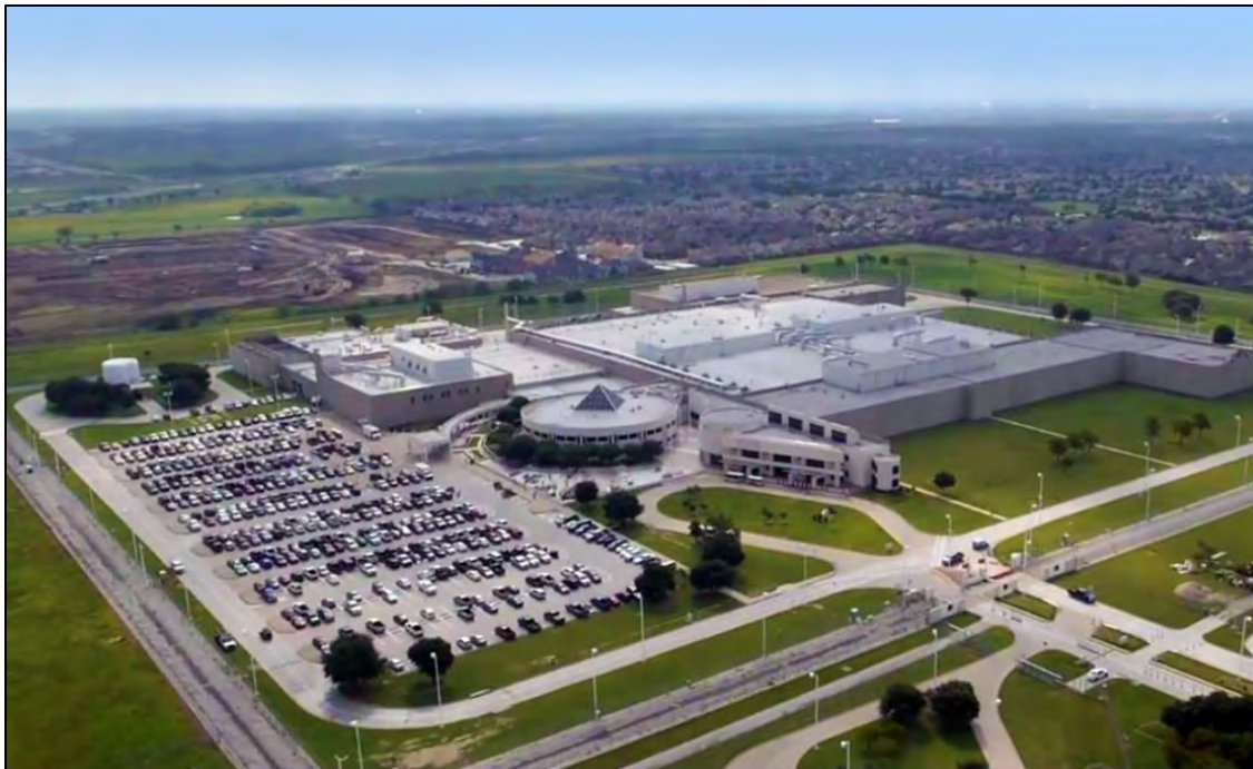
Figure 2.2-1: Western Currency Facility in Fort Worth, Texas
