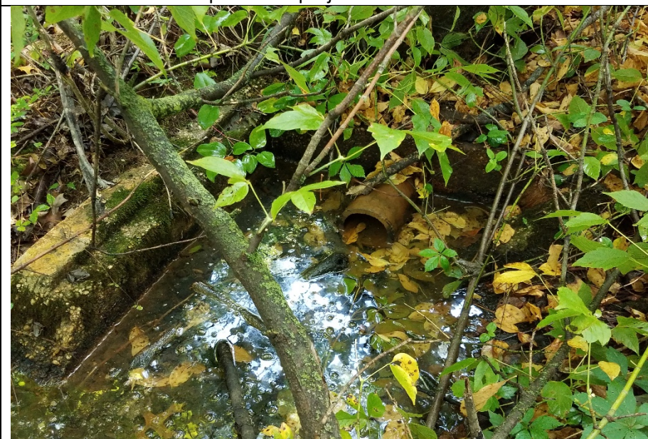
Wetland 1 – concrete headwall and terra cotta pipe at top of wet area
