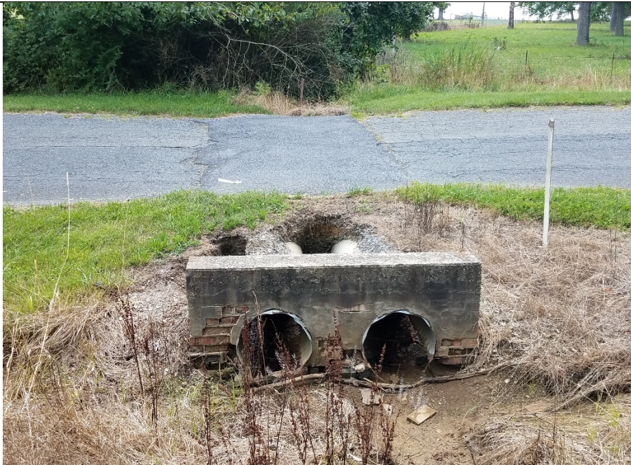
Culvert which drains WUS-4 and Wetland 4 under Poultry Road
