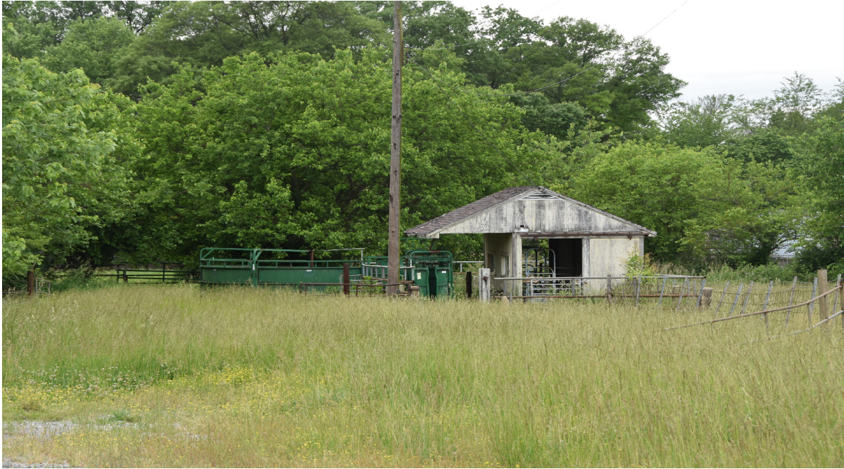
Photo 1 - Building 192G, Scale House, Central Farm, View of East Elevation, Looking West
