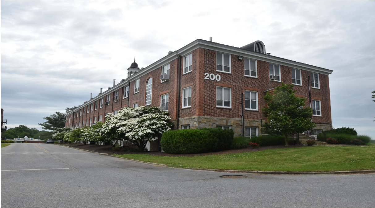
Photo 1 - Building 200, Main Laboratory, Central Farm, View of Northwest Oblique, Looking Southeast
