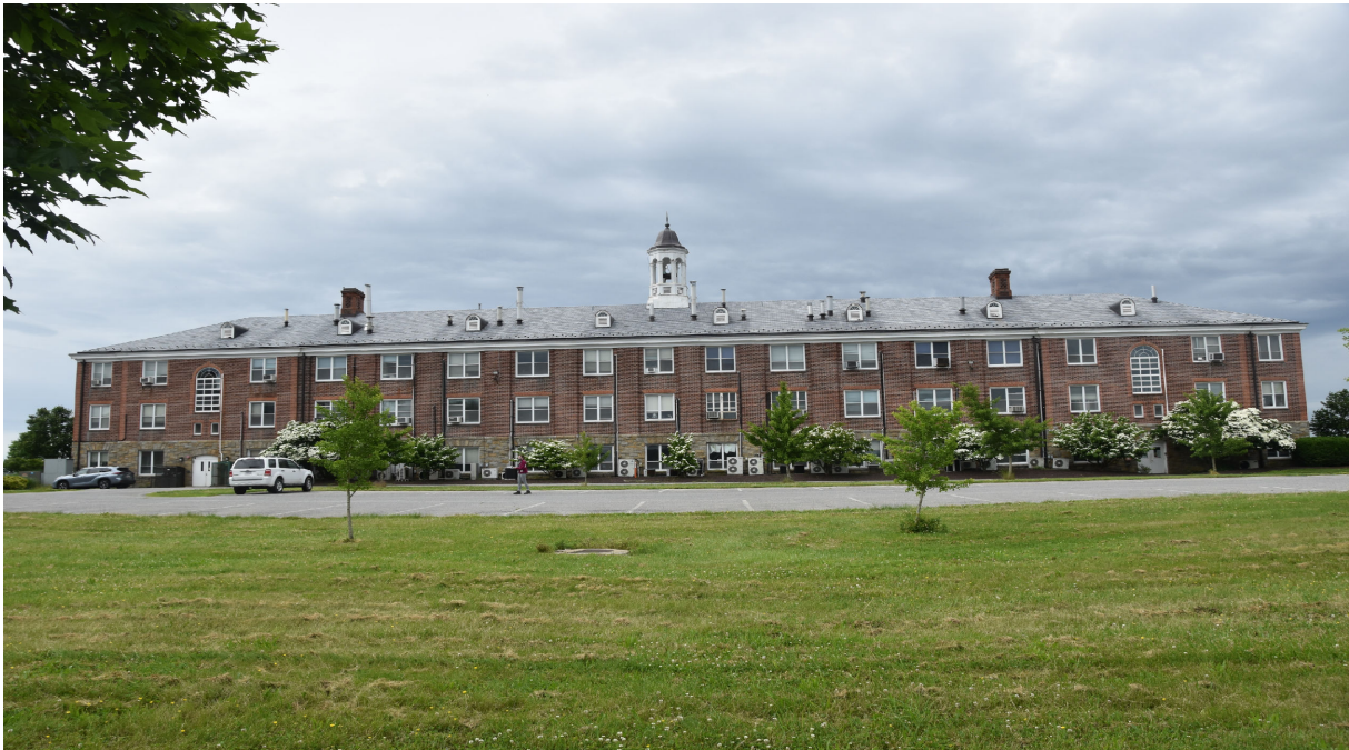
Photo 2 - Building 200, Main Laboratory, Central Farm, View of North Elevation, Looking South
