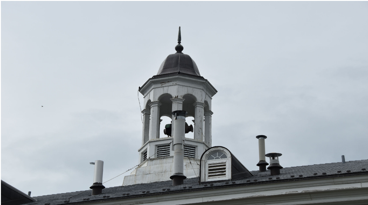
Photo 4 - Building 200, Main Laboratory, Central Farm, View of Cupola Detail, Looking Southeast
