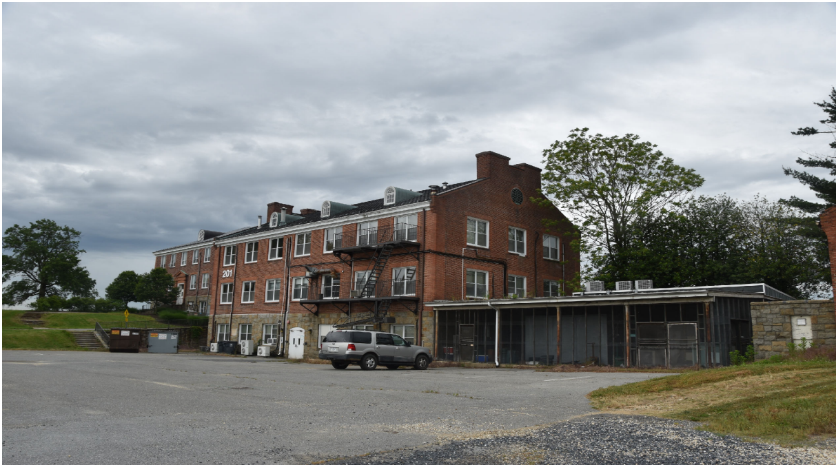
Photo 4 - Building 201, Small Animal Building (East), Central Farm, View of Northeast Oblique, Looking Southwest
