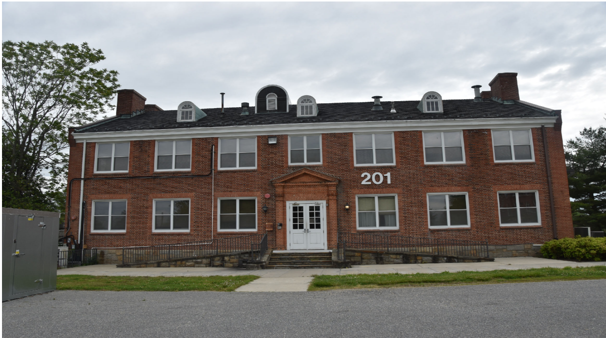
Photo 1 - Building 201, Small Animal Building (East), Central Farm, View of West Elevation, Looking East
