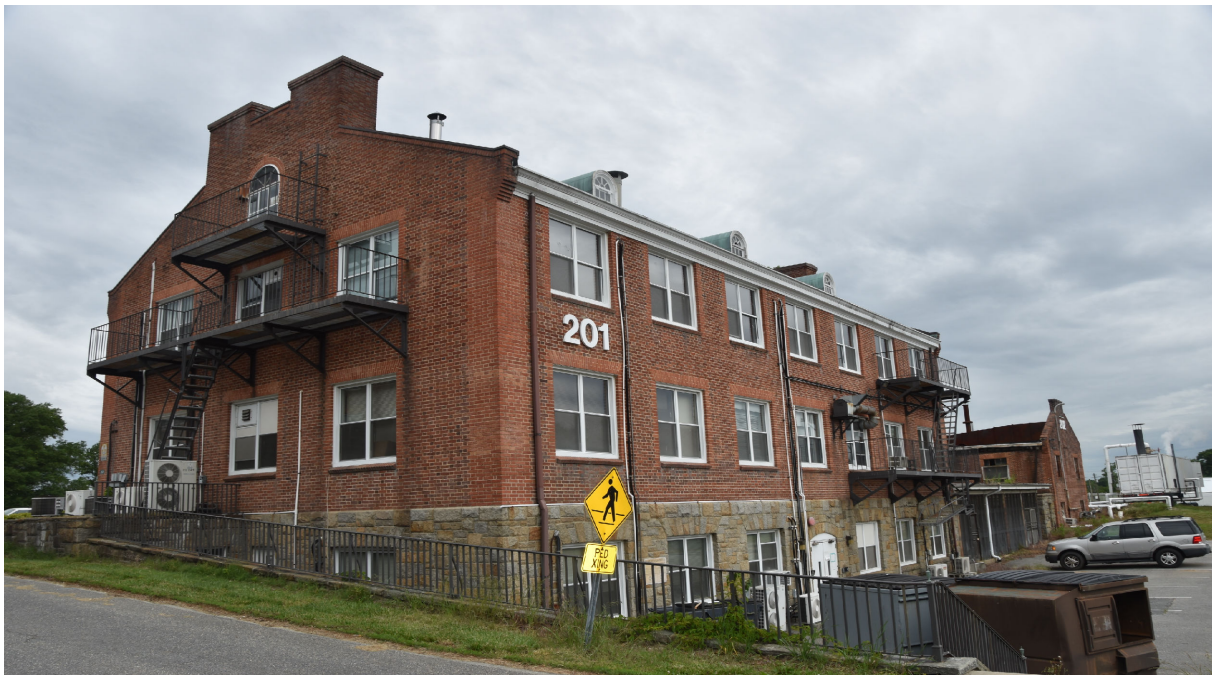
Photo 2 - Building 201, Small Animal Building (East), Central Farm, View of Southeast Oblique, Looking Northwest
