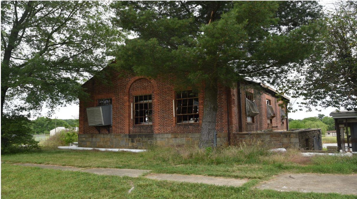
Photo 2 - Building 202, Boiler House, Central Farm, View of Southwest Oblique, Looking Northeast
