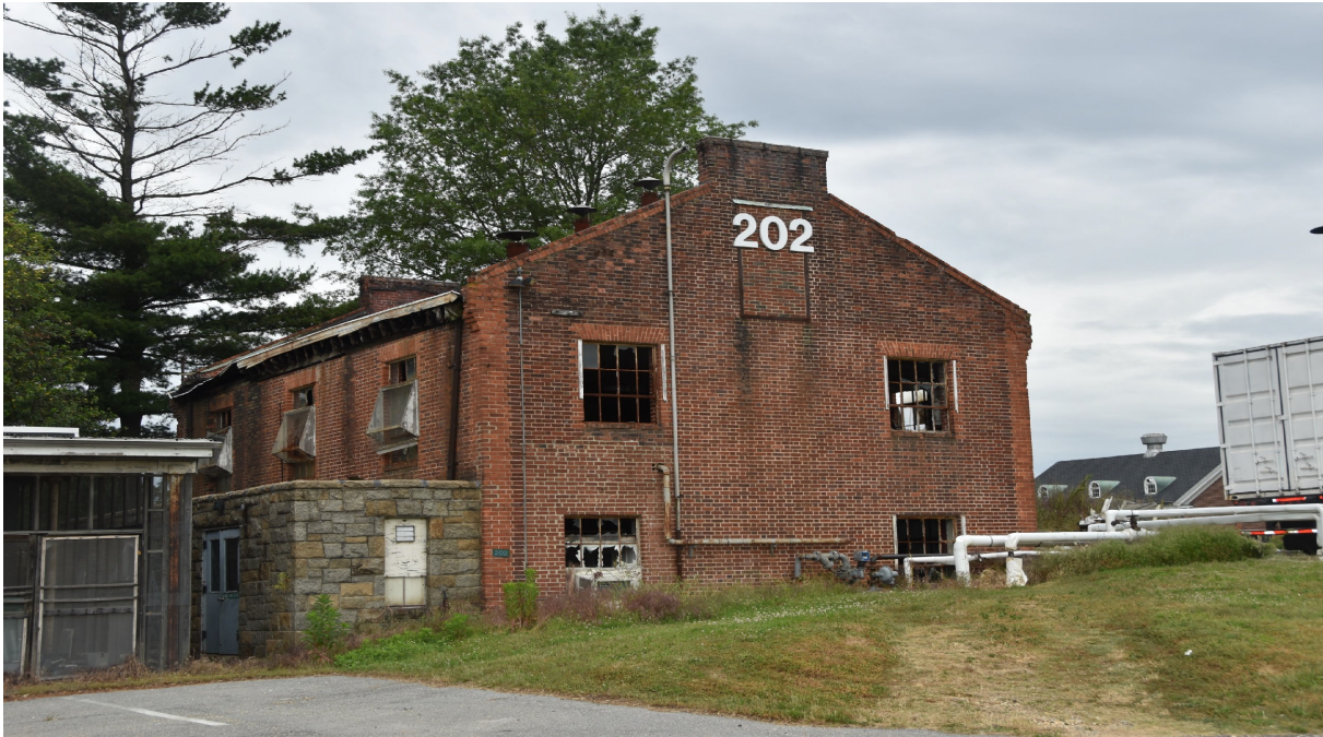
Photo 1 - Building 202, Boiler House, Central Farm, View of Southeast Oblique, Looking Northwest
