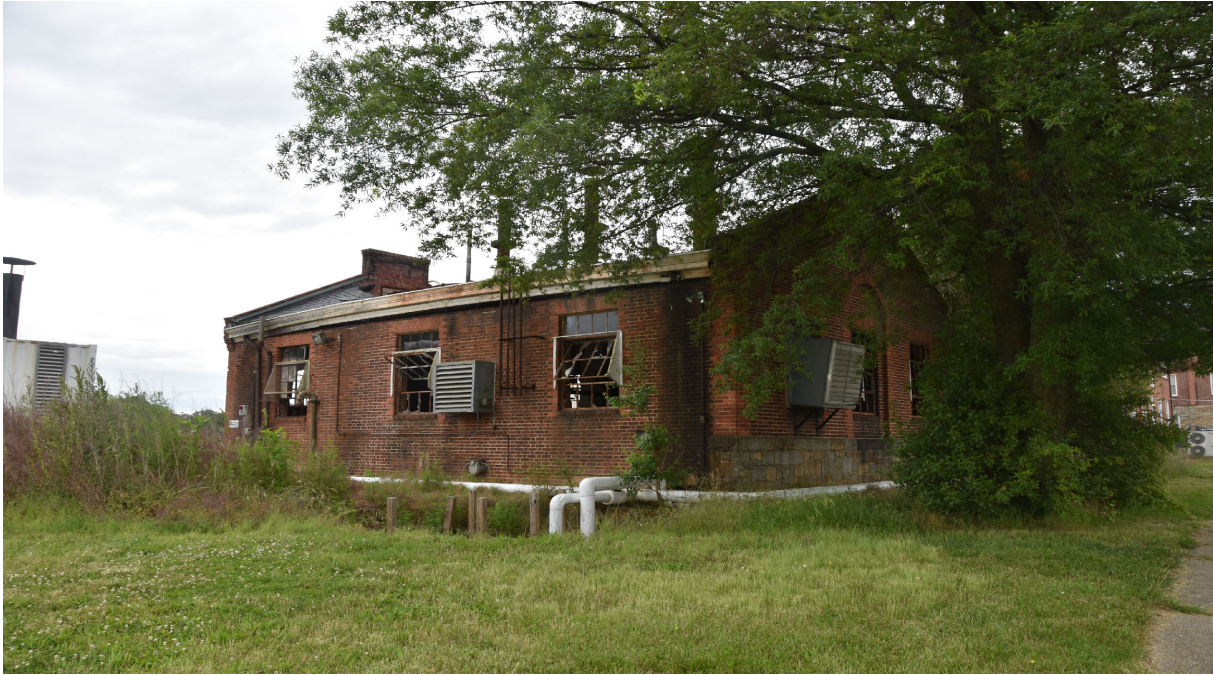
Photo 3 - Building 202, Boiler House, Central Farm, View of Northwest Oblique, Looking Southeast
