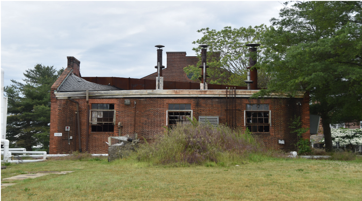
Photo 4 - Building 202, Boiler House, Central Farm, View of North Elevation, Looking South
