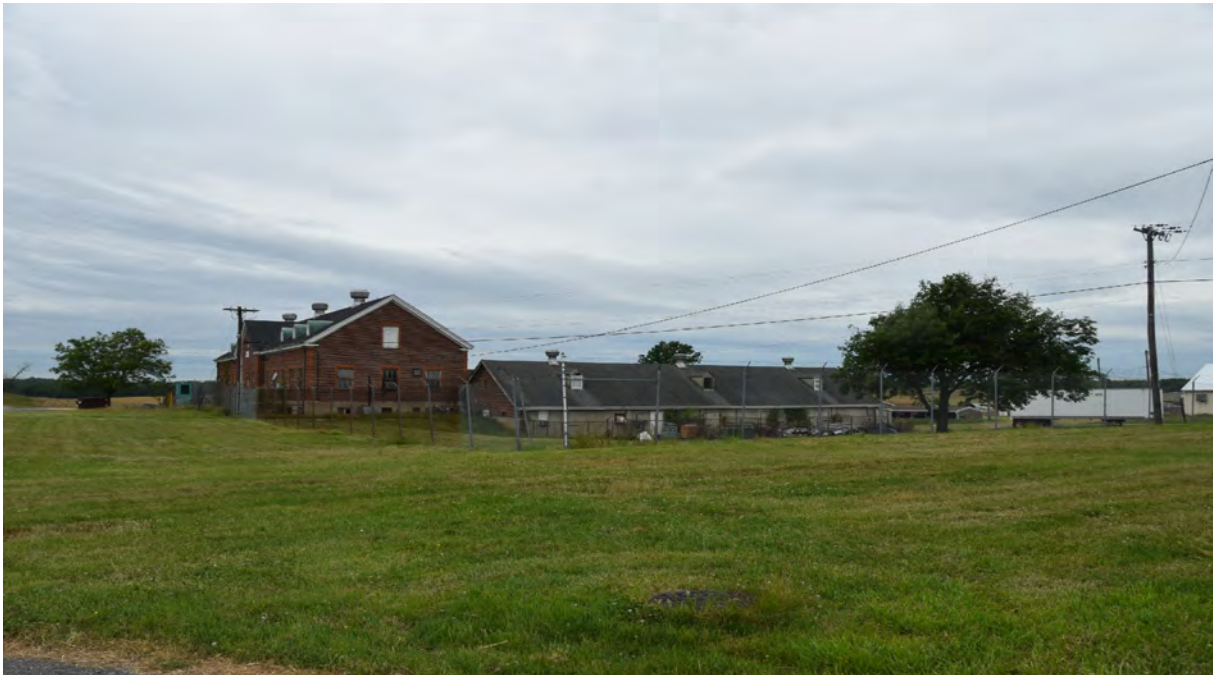
Photo 4 - Building 203, Large Animal Building, Central Farm, View of East Elevation, Looking West
