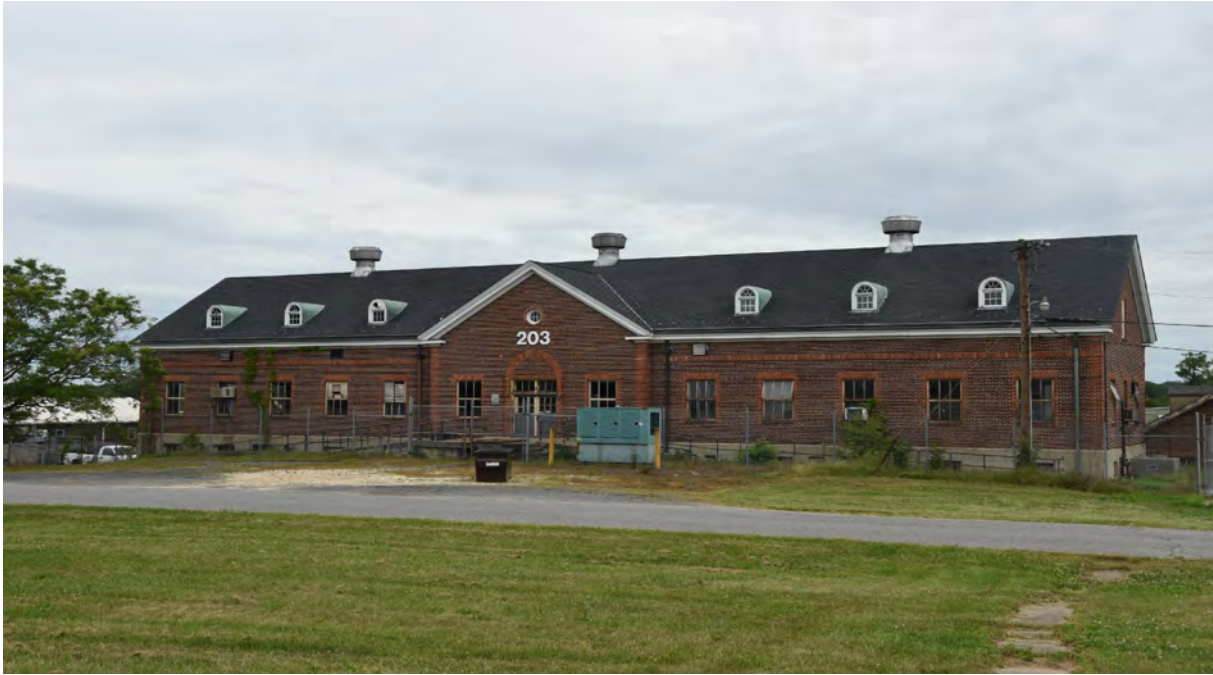
Photo 1 - Building 03, Large Animal Building, Central Farm, View of South Elevation, Looking North
