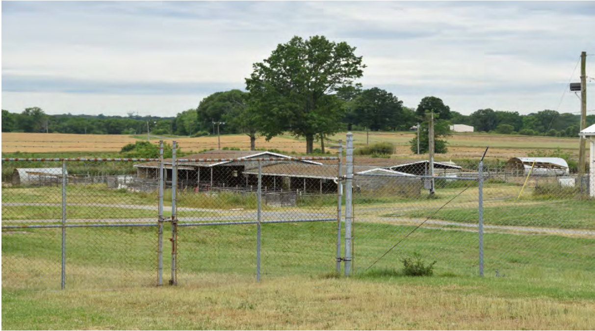
Photo 1 - Building 203A, Animal Shelter, Central Farm, Oblique view of South Elevation, Looking Northwest
