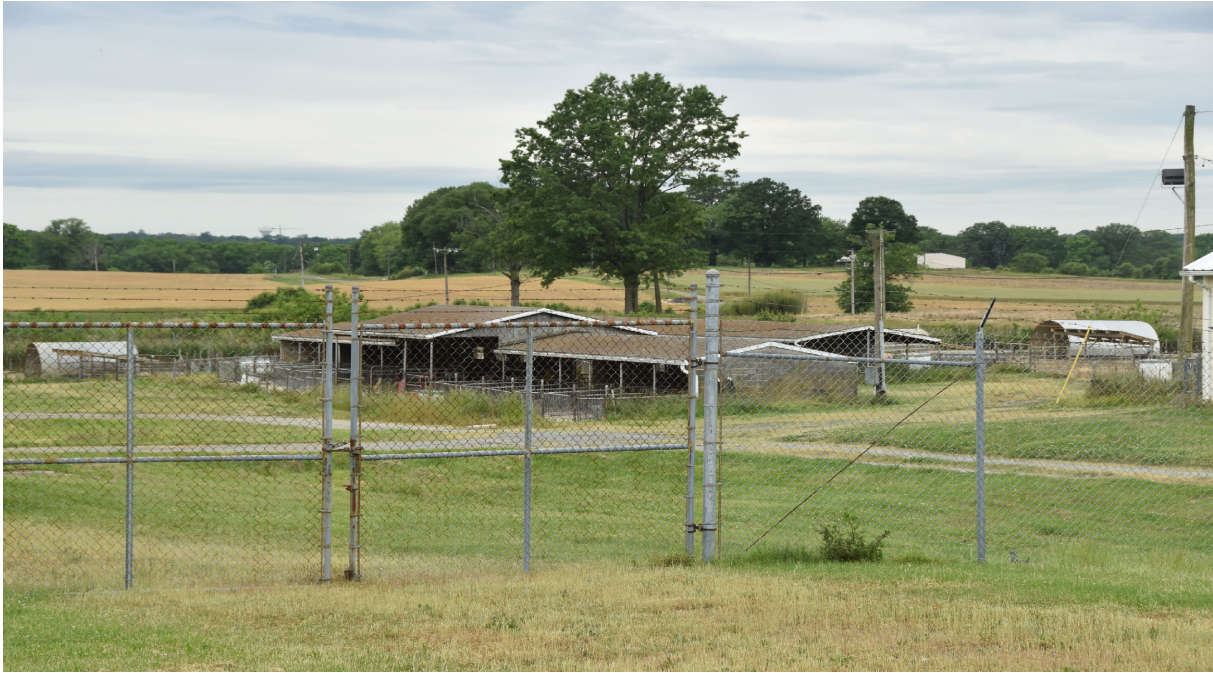
Photo 1 - Building 203B, Animal Shelter, Central Farm, View of East Elevation, Looking Northwest (Note: The shallow, side-gabled roof of Building 203B is right of field.)
