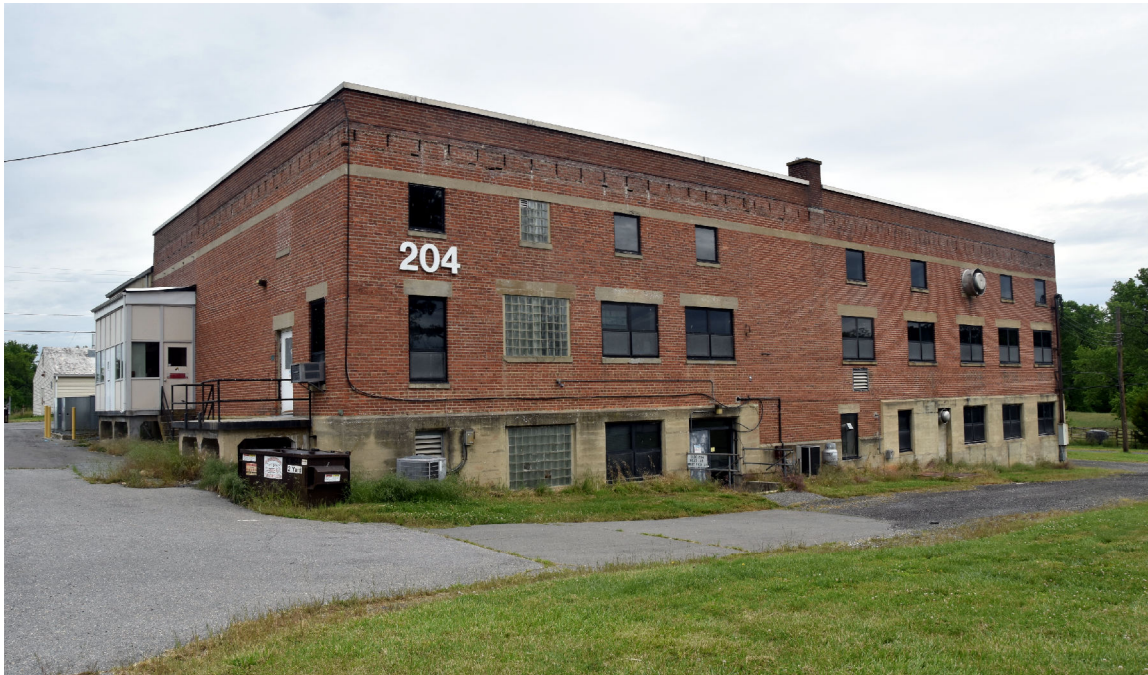
Photo 2 - Building 204, Meat Laboratory, Central Farm, View of South and West Elevations, Looking Northeast
