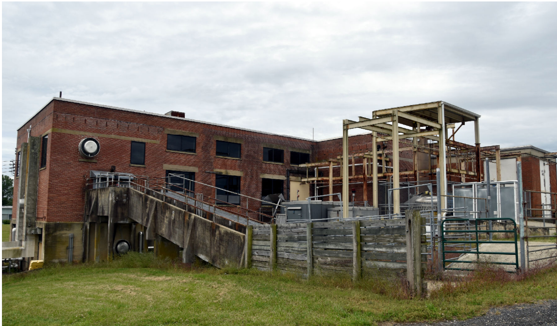
Photo 4 - Building 204, Building 204, Meat Laboratory, Central Farm, View of North Elevation, Looking South
