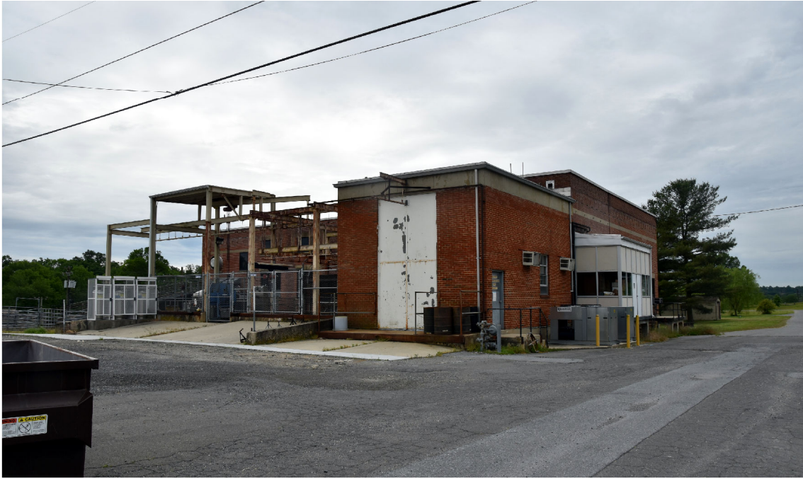
Photo 5 - Building 204, Meat Laboratory, Central Farm, View of North and West Elevations, Looking Southeast
